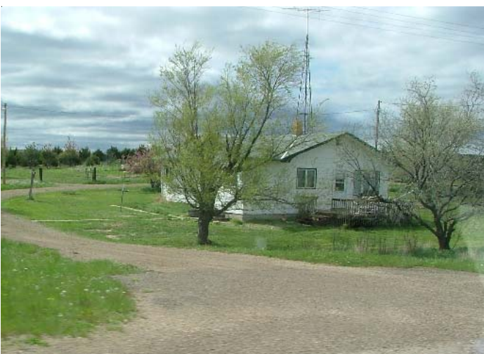
Fuel breaks, survivable space, Firewise construction and deciduous vegetation make this house defendable from wildfire.
