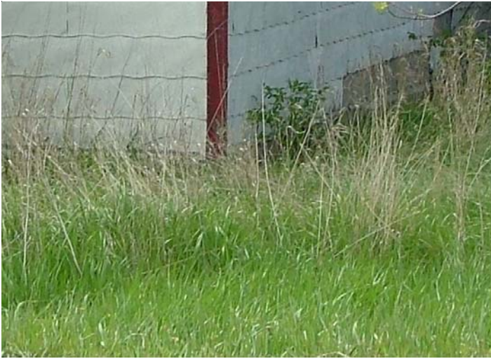
Uninterrupted fuels can allow a fire to spread to a structure.
