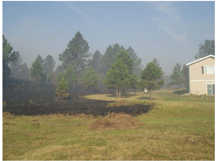
Firewise landscaping helped this structure to survive wildfire.
